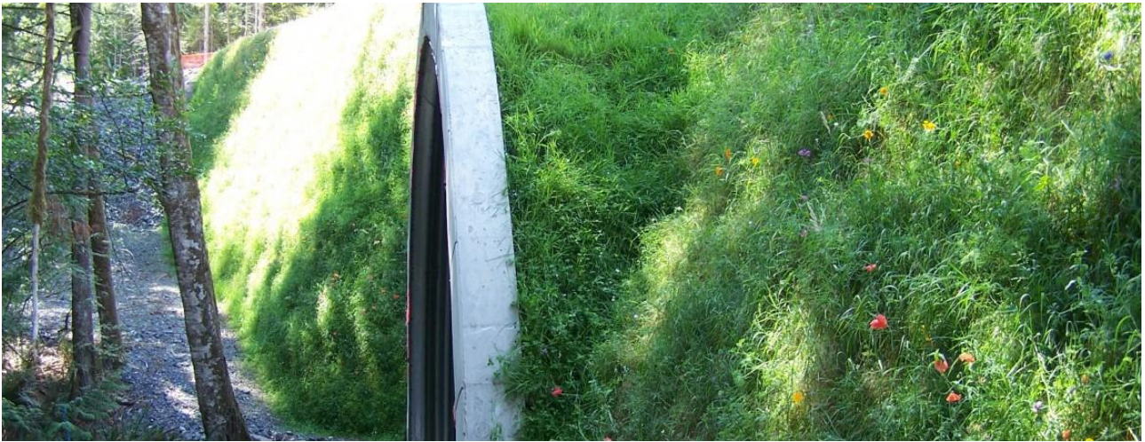
Image 4.30: Vegetated green wall retaining solution, following vegetation growth
