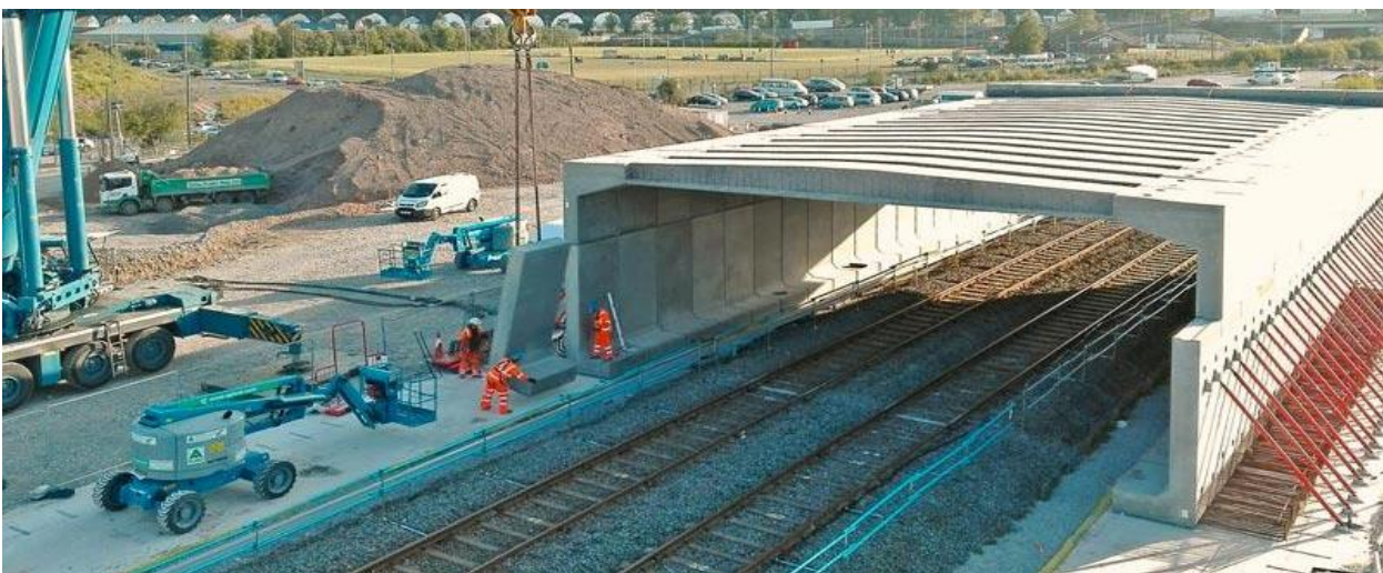
Image 4.19: Example of segmental precast reinforced concrete porta frame structure over rail
