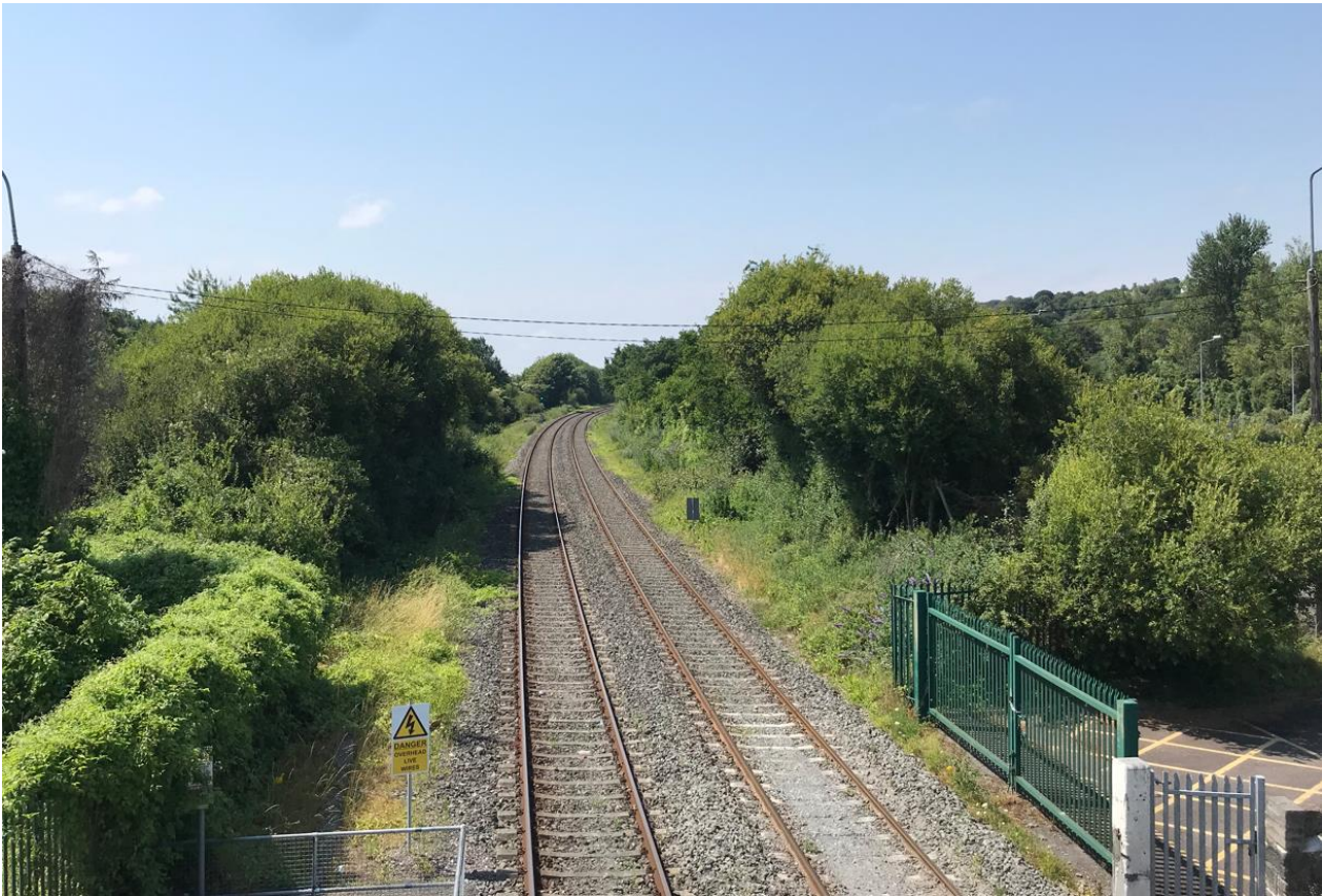
Image 4.10: Irish Rail tracks – looking west from Little Island station
