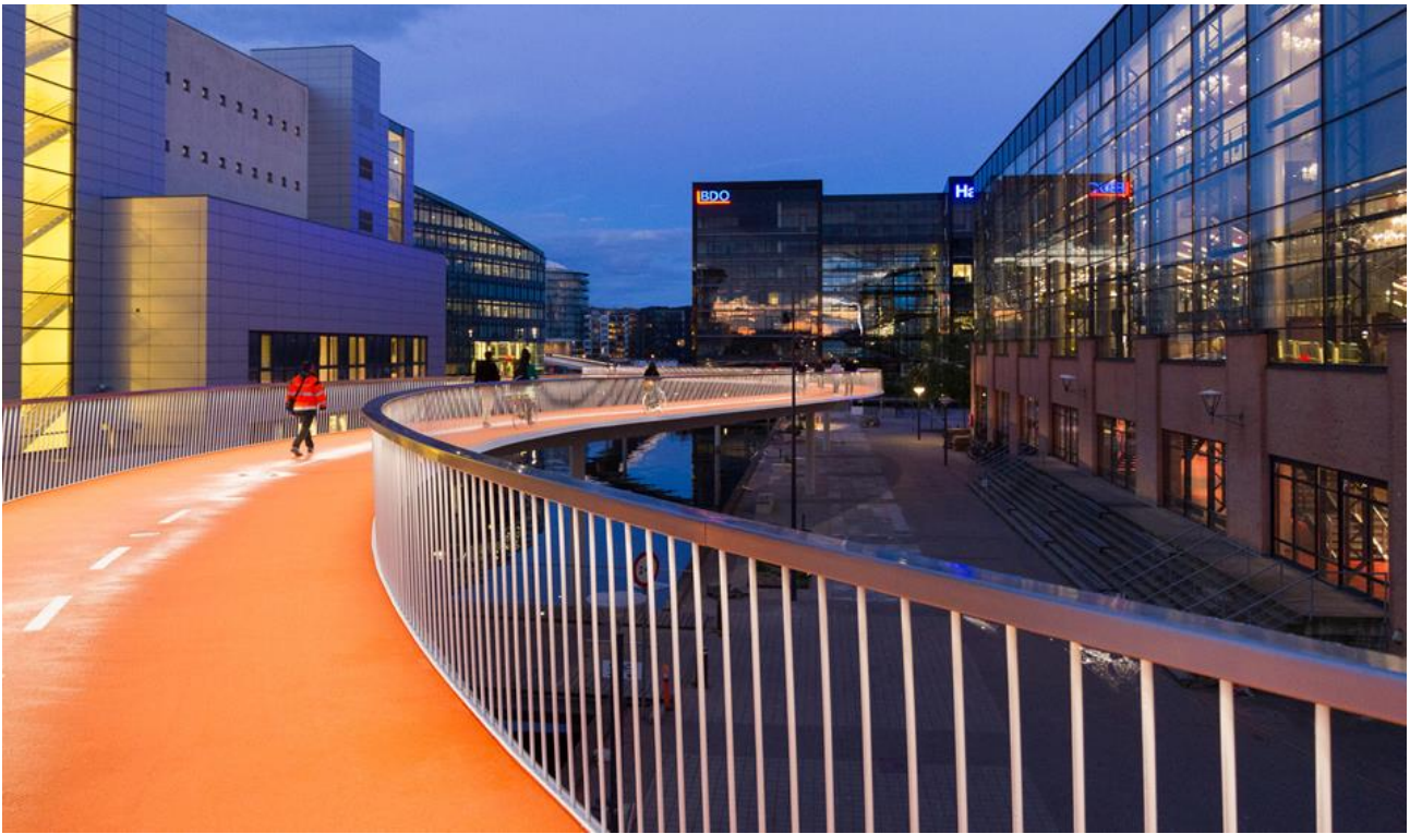
Image 4.26: Parapet type with vertical parapet infill
