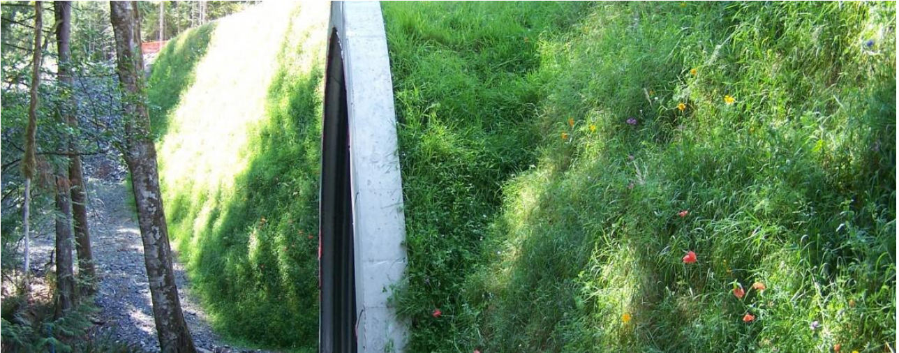
Image 4.24: Vegetated green wall retaining solution, following vegetation growth
