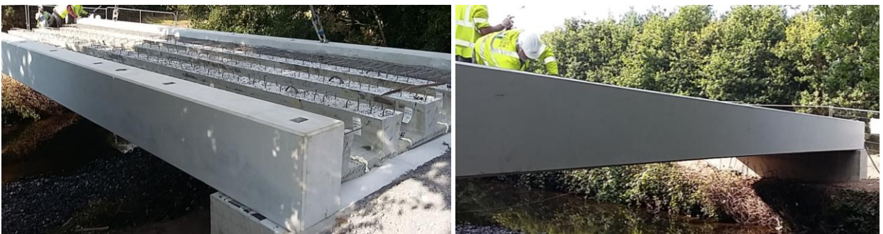
Image 4.22: Precast prestressed concrete bridge beams for approach ramp elevated structure (as proposed for the southern approach ramp)
